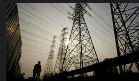
WEST TO EAST ELECTRIC POWER
